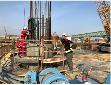
Installation of test pile
